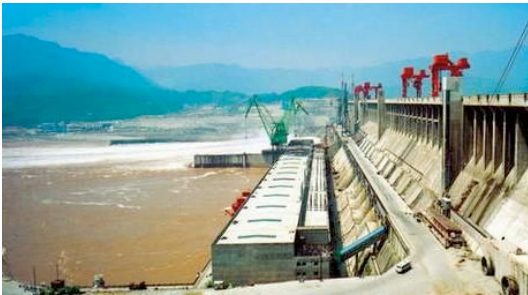
A side view of the dam
